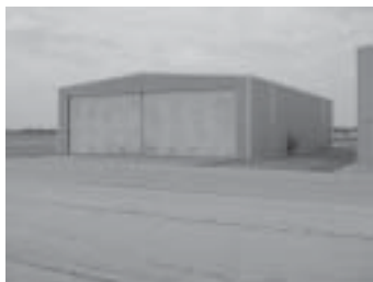
Overhead doors face secured entrance
